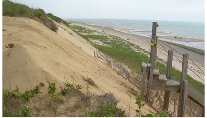
Eroded grades re-connected.
