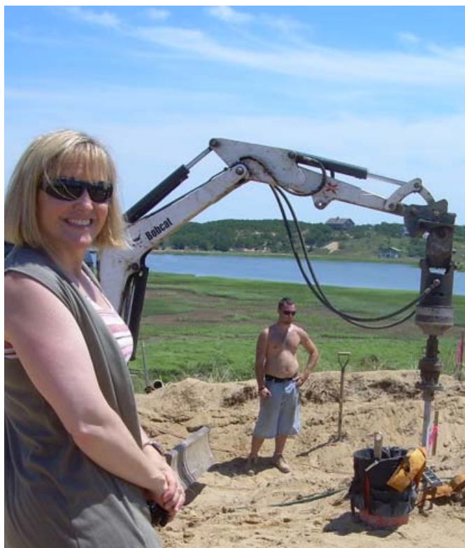
Joy Cuming watches the installation process.
