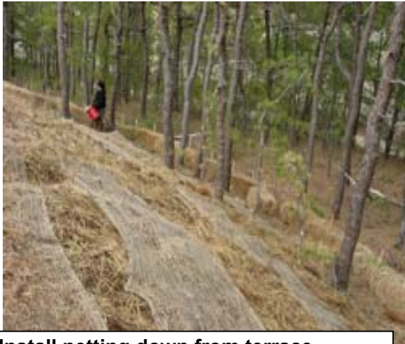
Install netting down from terrace
