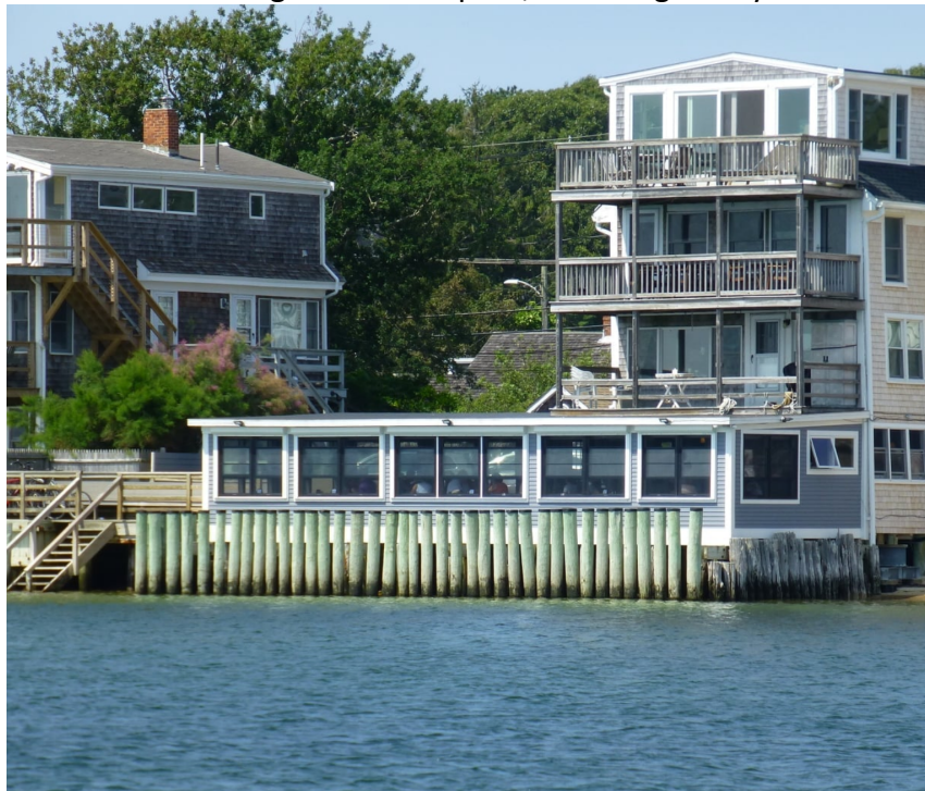
Image above showing conditions at grade after nearly 20 years of use: No erosion; no accretion; no destabilization and no change in vertical piles, following nearly two decades of storms.
