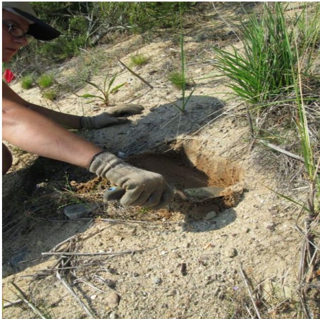
Images by G. Peabody. 24” shelving, using a trowel, forms downslope berm.
