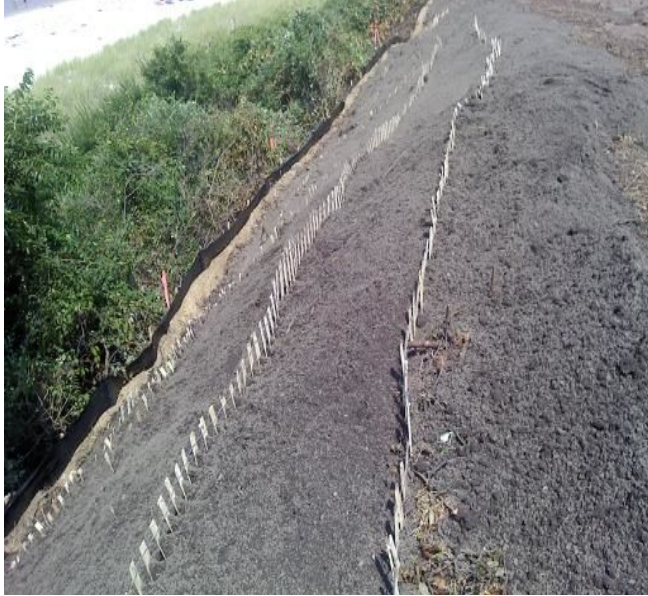
Images by G. Peabody. Stages in the bioengineered, slope stabilization process.
