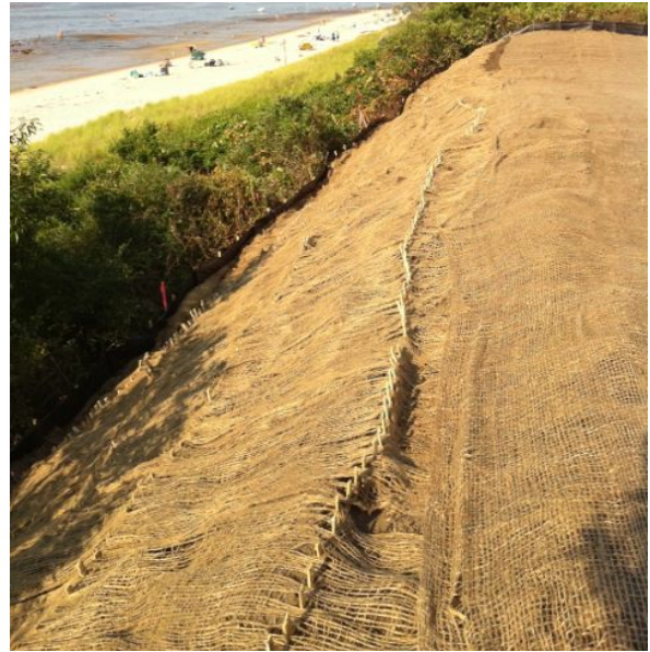
Images by G. Peabody. Stages in the bioengineered, slope stabilization process.
