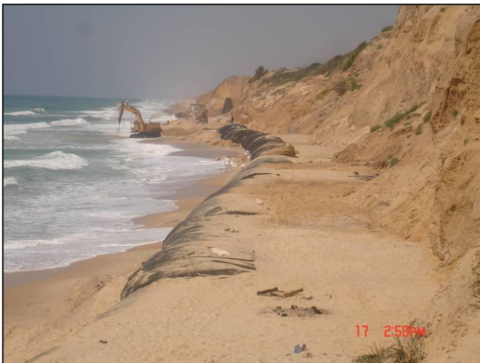
Figure 7 –Geotextile tubes at the base of the Ashkelon Cliffs, Israel.
