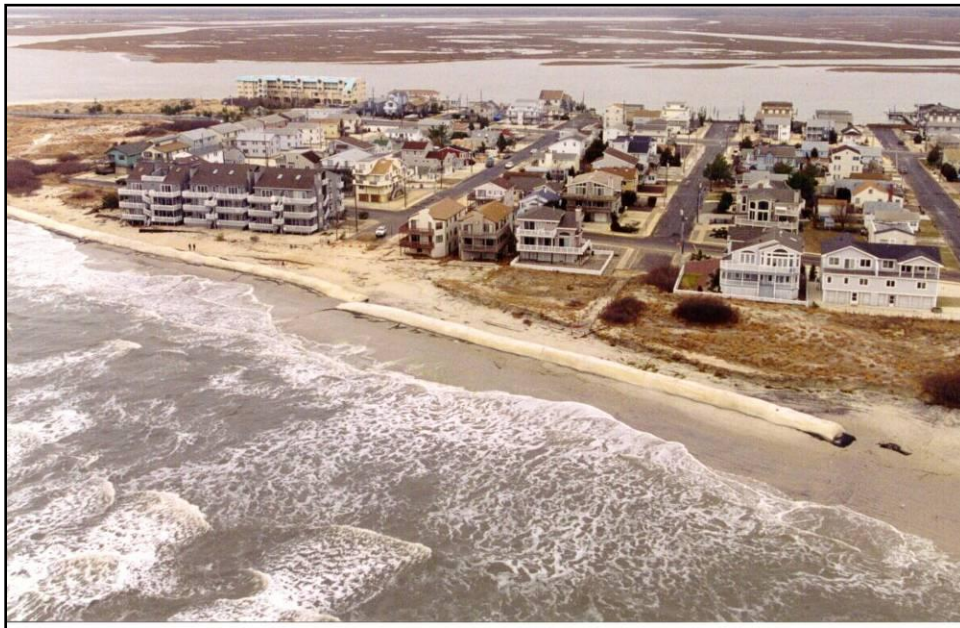
Figure 6 – Aerial view of geotextile tubes in Sea Isle City, NJ, 1998.
