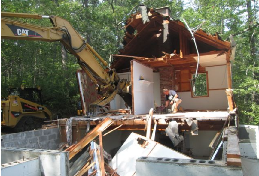
Above image by Safe Harbor. Shows removing copper pipe.
