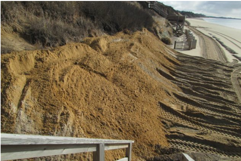
Nourishment is then spread up the lower bank.
