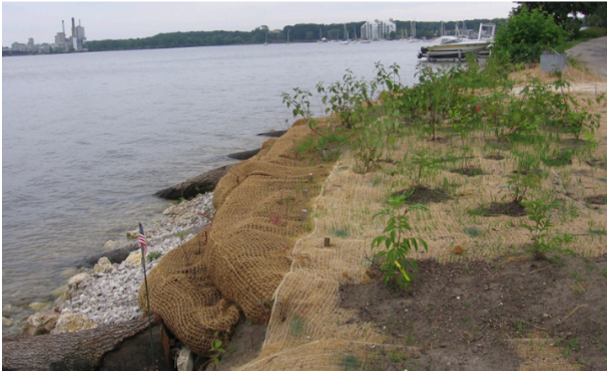
Fully “Ballasted Coir”, in freshwater, with native plantings. Muskegon Lake Watershed.
