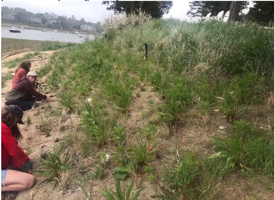
Image G. Peabody, stone ballasted coir with nourishment and vegetation 1 st year
