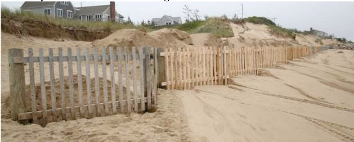
Image above: Large, treated posts require excavation to support typical Bayside sand drift fence. This alternative is now being re-evaluated in some communities.
