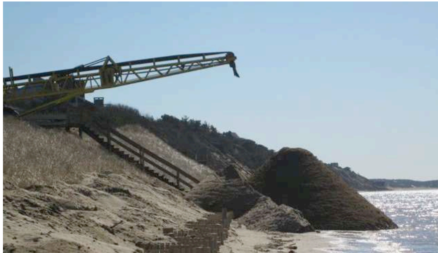
Image above: Conveyor being used to deliver sand to toe of bank.
