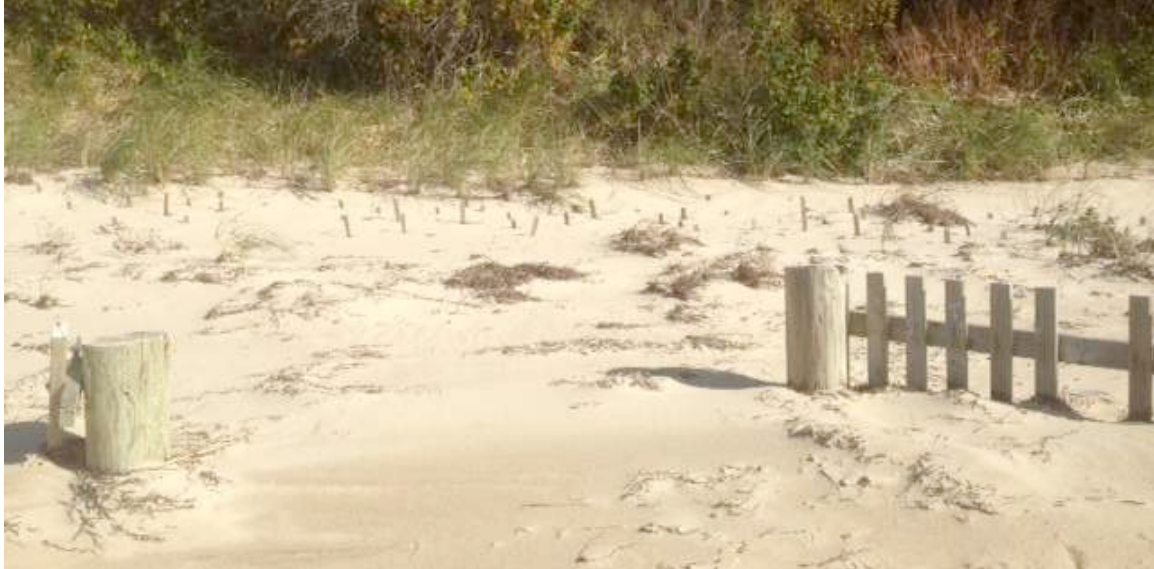
Image above by G. Peabody: sand accumulations seem unaffected by drift fencing
