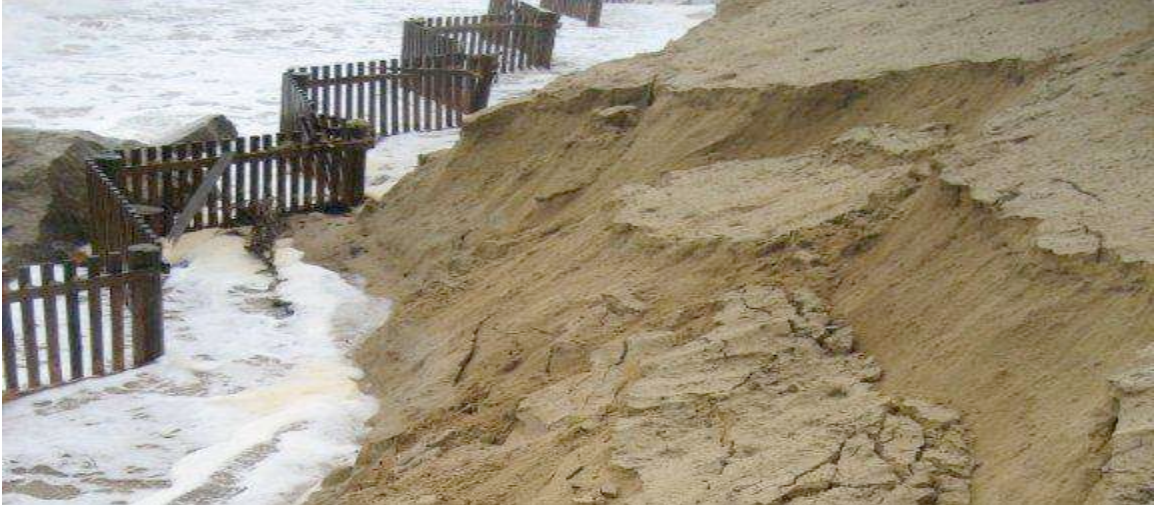
Image above: Drift Fence may restrict overwash outflow, contributing to outwash of sand.
