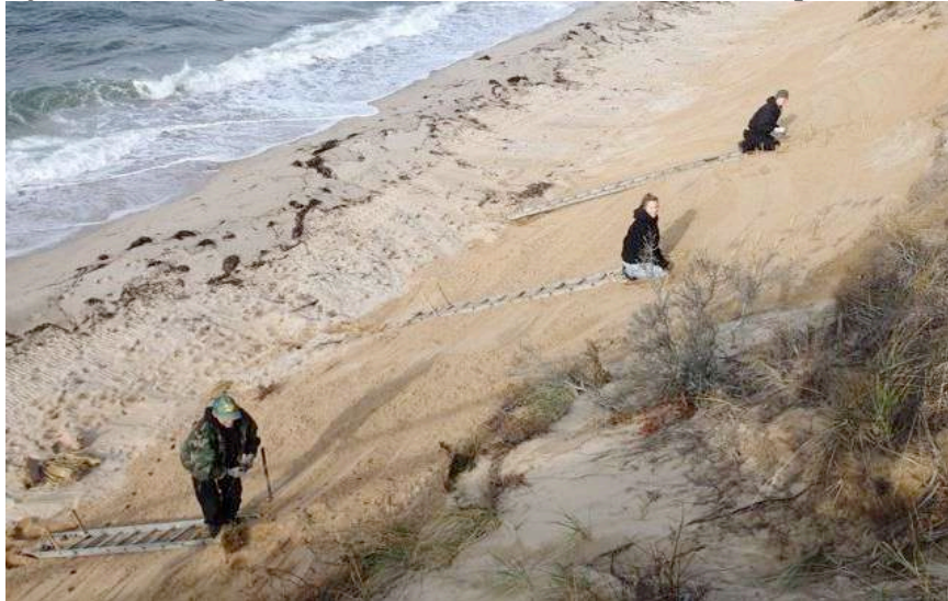
Using ladders to plant protects new nourishment by avoiding destabilization
