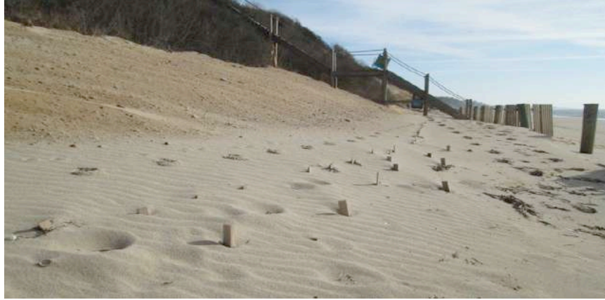
Biomimicry collection systems can be raised to collect more sand.
