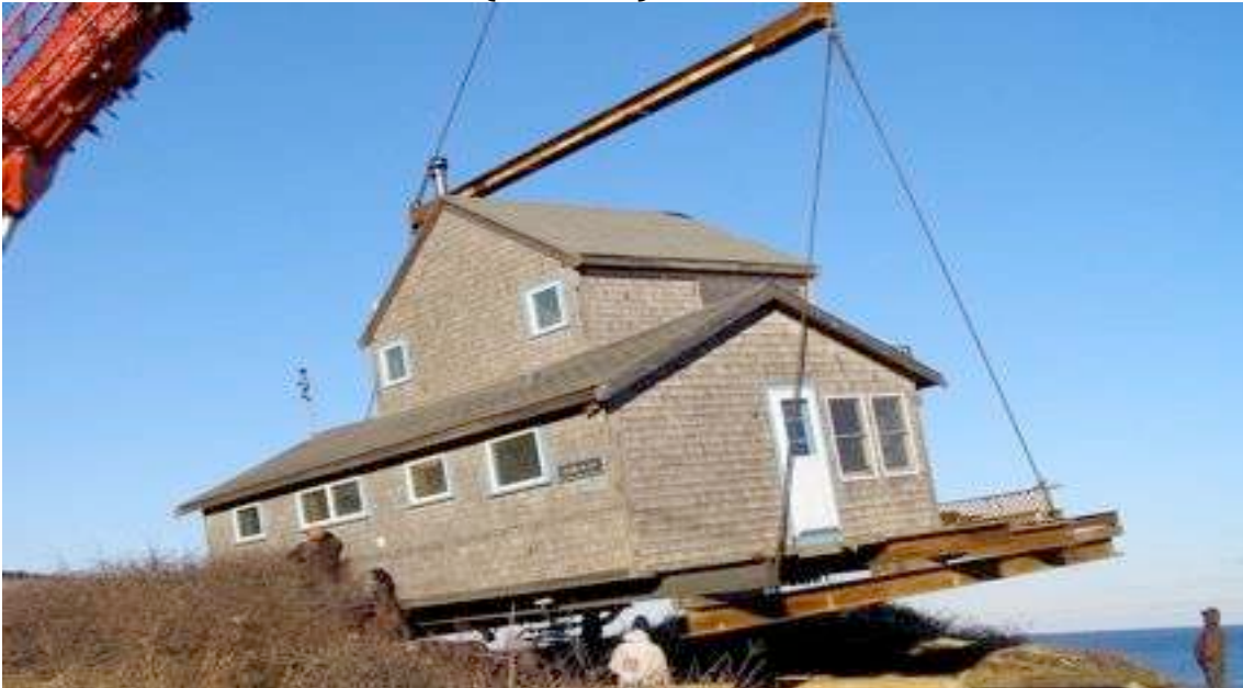
Image above by G. Peabody: Relocating a residence away from a coastal bank. Costs: Significantly less than rebuilding; Permitting often facilitated by Municipalities; Stabilize removal site. Consequences: 100' = 30-40 years.
