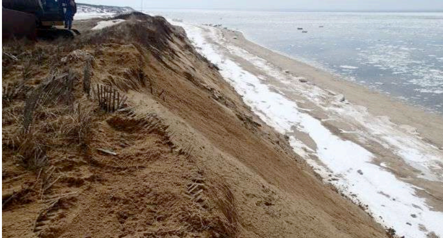
Image above shows more sustainable, full bank nourishment.
