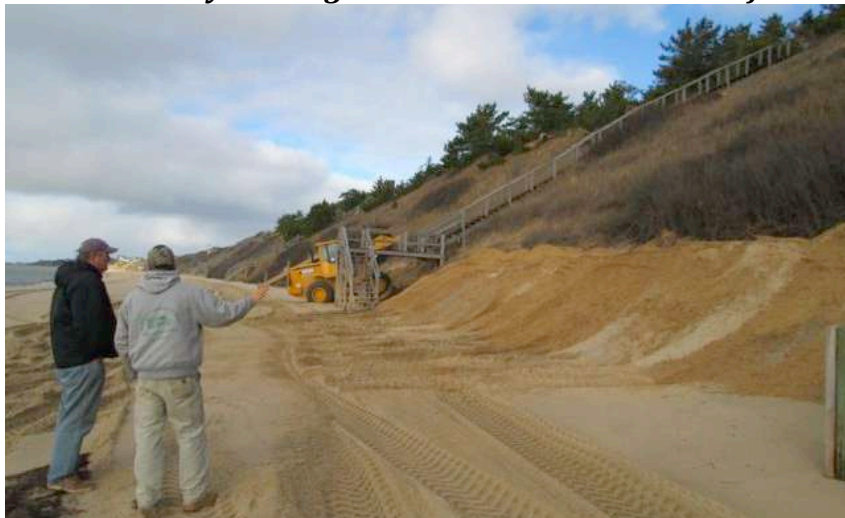
Image above: Sand renourishment at toe of bank requires beach access.
