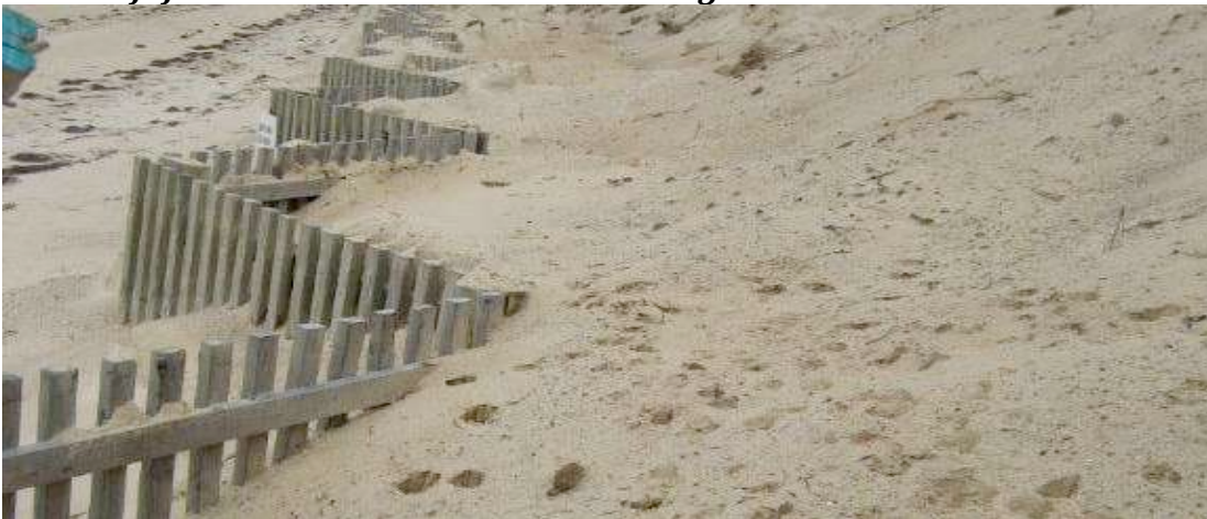
Image above: Drift fences also require sand nourishment and beach grass planting. Nourishment and vegetation often require annual replacement.
