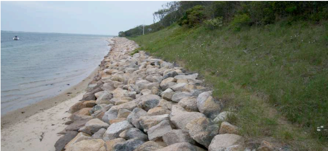
Image by G. Peabody: Revetments may interrupt bank to beach sediment flow.
